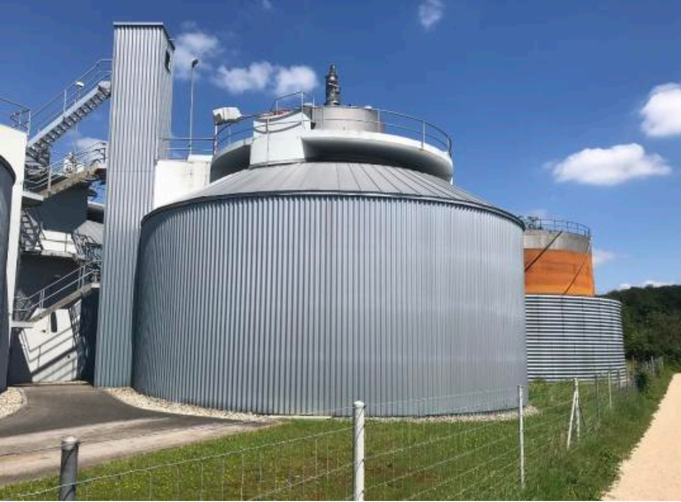
Swiss Waste Water Treatment Plant Summer 2019
