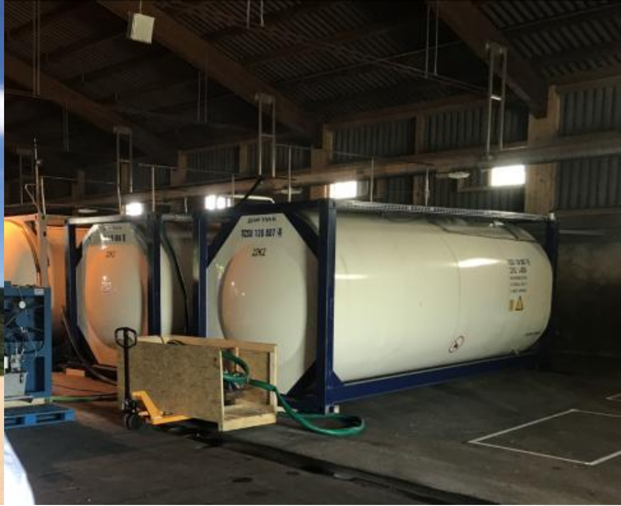
Demo at Waste Water Treatment Plant Summer 2019
