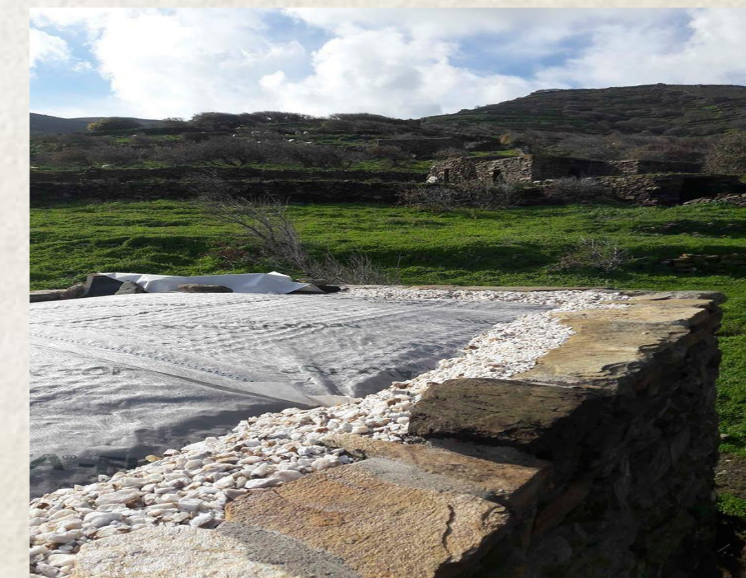
Waterproof roof for rainwater harvesting
